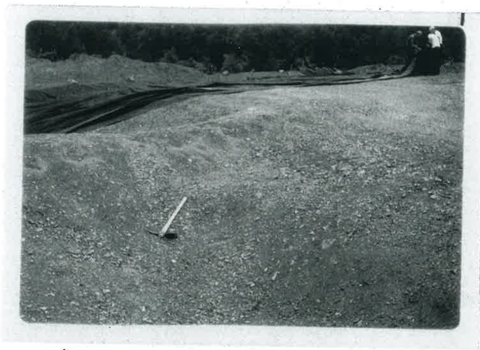
Figure 9. This view shows sewing and fitting of fabric on the small leach pads.
