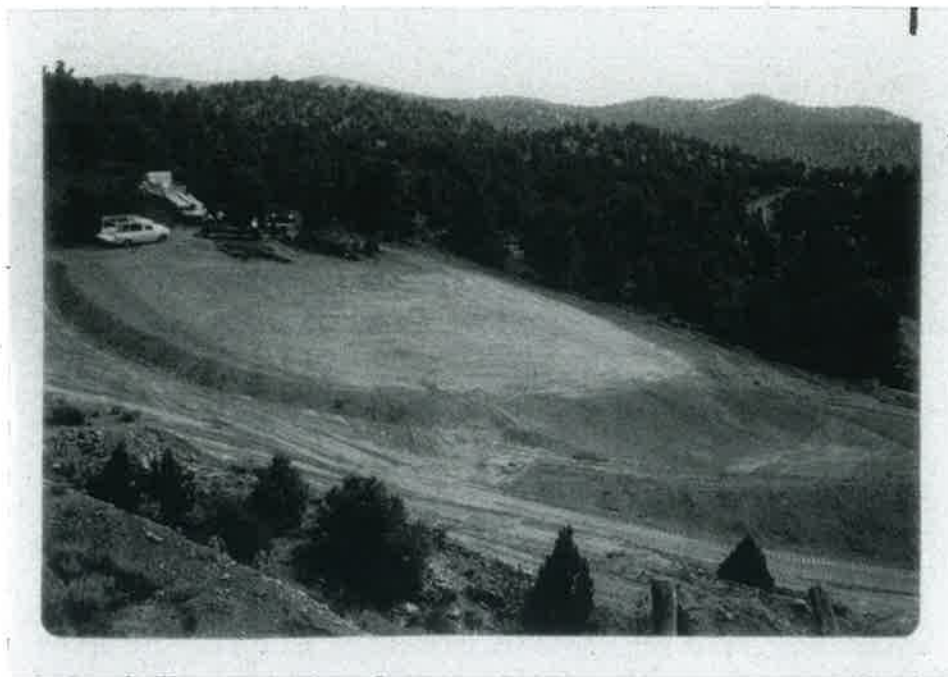
Figure 6. View of the 5000 ton pad area just as mat is starting to be unrolled. Notable features are the pond area with uncompacted berm, and the small uncompacted peripheral berms which direct solutions into the pond. Not so obvious is that the pad area is slightly crowned so solutions flow to the left and right berms as well as straight into the pond. Road at extreme right can be keyed to Figure 3.
