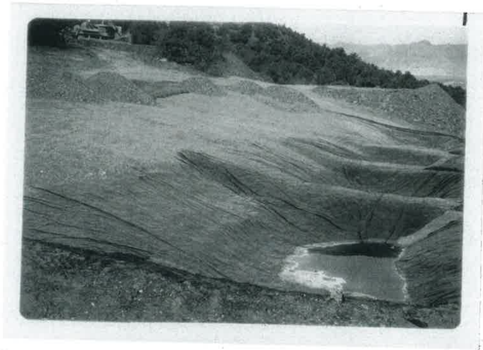
Figure 7. View looking west across the four small pads. The pads have been completed, and a 2" gravel cover has been applied. First and second lifts of the 5000 ton pad are shown in background.
