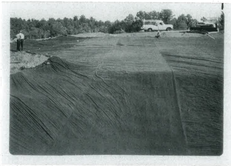
Figure 10. View looking south, across the pond to the 5000 ton leach pad. The sewn joints and some of the folds are visible.
