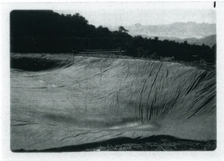
Figure 5. View looking west at the pond for the 5000 ton leach, showing the north berm. This photograph was taken following lining with fabric but before spraying. Rain is responsible for the standing water. The sewn joints can be seen on 15 foot intervals, along with several folds in the cloth which caused some sealing problems. The berm shown, consists of 10 feet of uncompacted fill.
