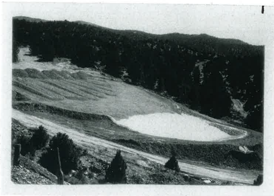
Figure 14. View showing the 5000 ton pad as the protective cover is being applied. The 2" gravel cover was placed by being dumped from an end-loader bucket and hand-raked. The 1-2 ft layer of 3-4" rock is being spread with a dozer. This view is taken from the same location as Figure 3.
