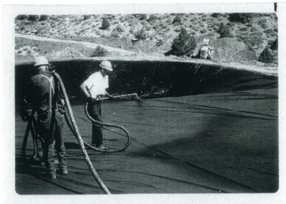
Figure 12. The asphalt was sprayed onto the pad as a brown water emulsion, which rapidly turned black as it dried. Three men were required to handle the hose. Occasionally the nozzles would plug due to the asbestos suspended in the asphalt; eventually we switched to a flattened piece of 3/4" pipe. Pressure for spraying was supplied by pressurizing the delivery truck.
